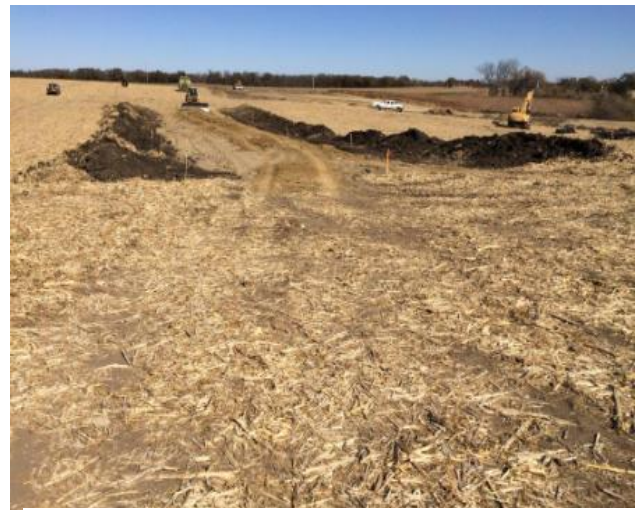
During construction of water and sediment control basin
